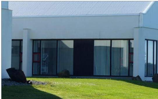
GARDEN CENTER Montijo BIG DUCT + T FRESH
