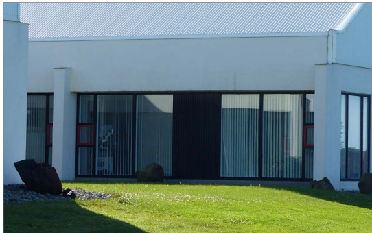
GARDEN CENTER Montijo BIG DUCT + T FRESH
