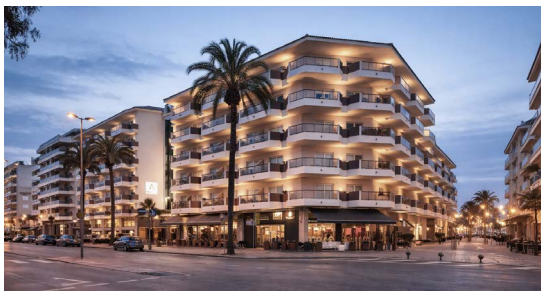
HOTEL PROMENADE Pineda de Mar CHILLER 240KW MODULAR
